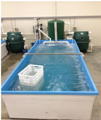
Holding (Stabling) Tank
