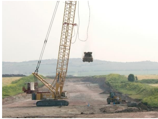
Figure 1.10 Technique compactage dynamique
