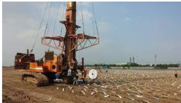
Figure1.13 Installation des drains
