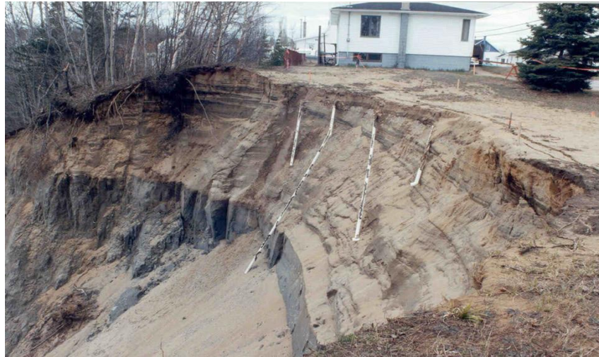
Figure 1: water infiltration into the soil due to a leaching field, (The Ministry of Public Security, Government of Quebec, 2017).
