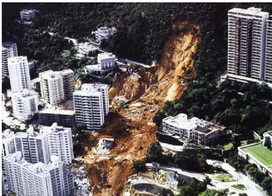
Figure 10: Shan Road landslide, Hong Kong, 1972, (Robert , et al., 2007).
