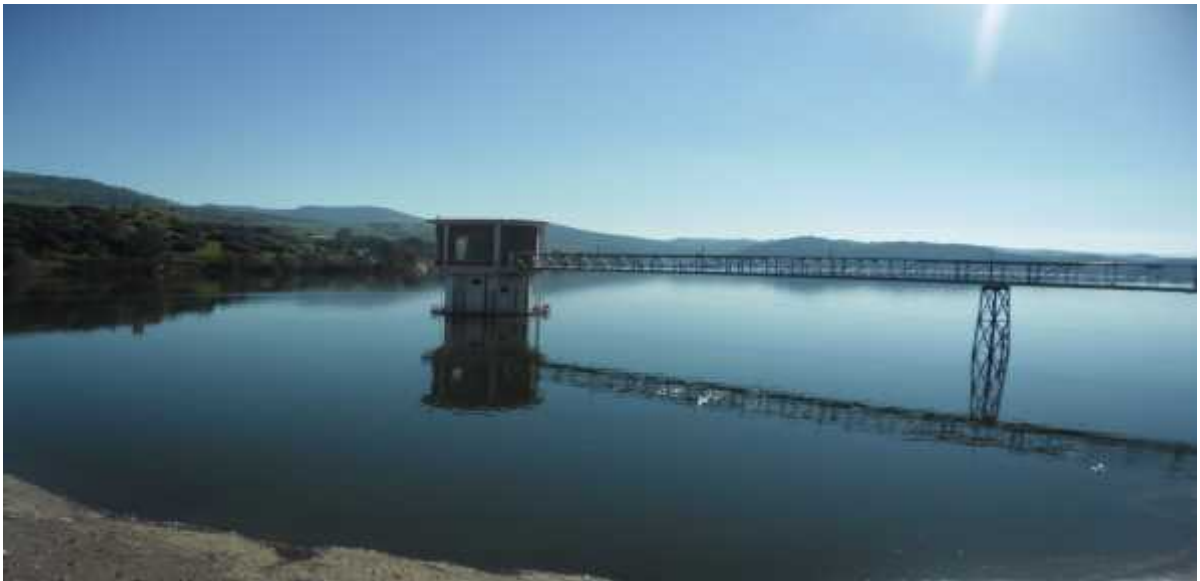
Figure n° 02: Photo du Barrage Ghrib (source: Azizou; Madani ;2015)
