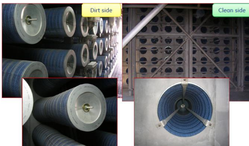
Figure II-9: Filtre auto-nettoyant
